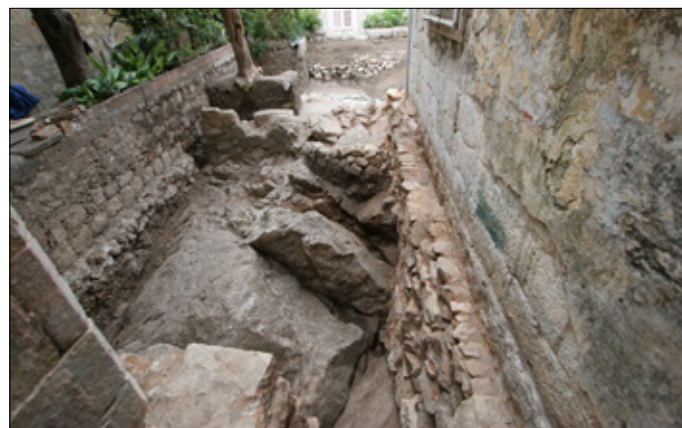
Samostan sv. Marije od Kaštela u Dubrovniku The Convent of St. Mary of Kaštel in Dubrovnik (foto: B. Milošević, 2008, Omega engineering d.o.o. Dubrovnik)
